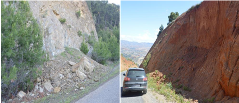
Figure 1 : The photos depict landslides threatening roads in the Boudinar basin
